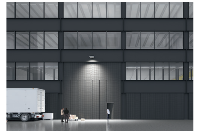
The huge sliding door makes it possible for trucks to get in and out
