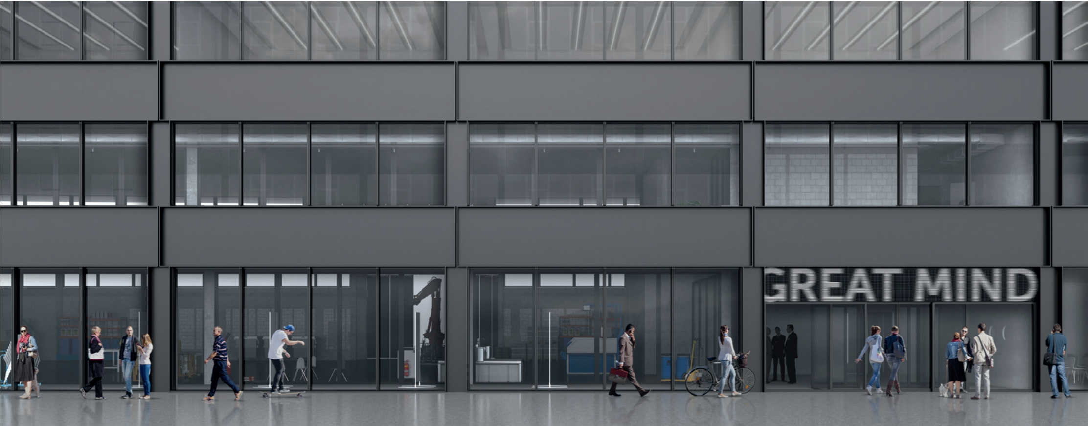
The new SIPBB building is certified to the Minergie-P standard
